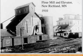
Why are they called elevators? Grain is lifted in order to load it into railroad boxcars. Conveyors lift grain to an overhead system of belts and chutes that carries it into different storage bins. From the high storage bins, grain drops by gravity into waiting railroad cars.
